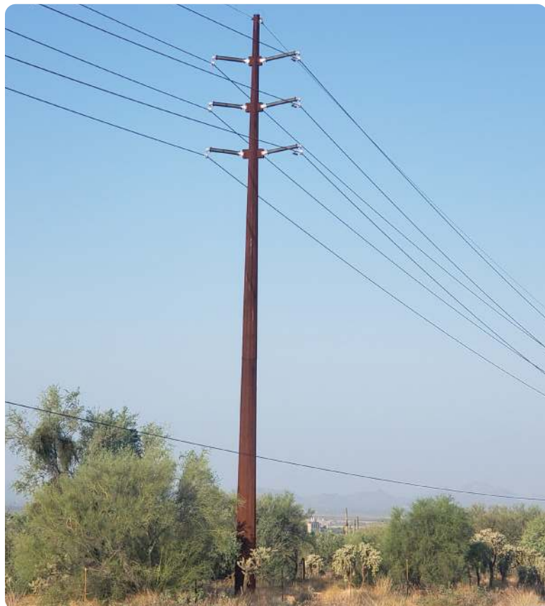
115 or 138kV Double Circuit Tangent Steel Monopole
